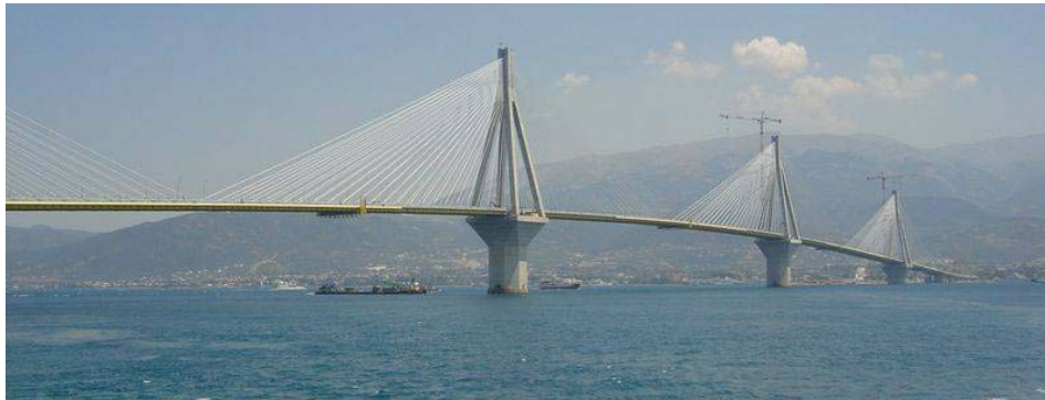
The bridge Rion, in Greece, where Citilog recently deployed its incident detection solution
