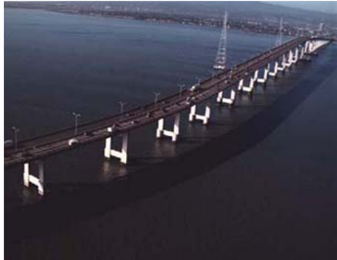
Figure 1 – San Mateo Bridge
